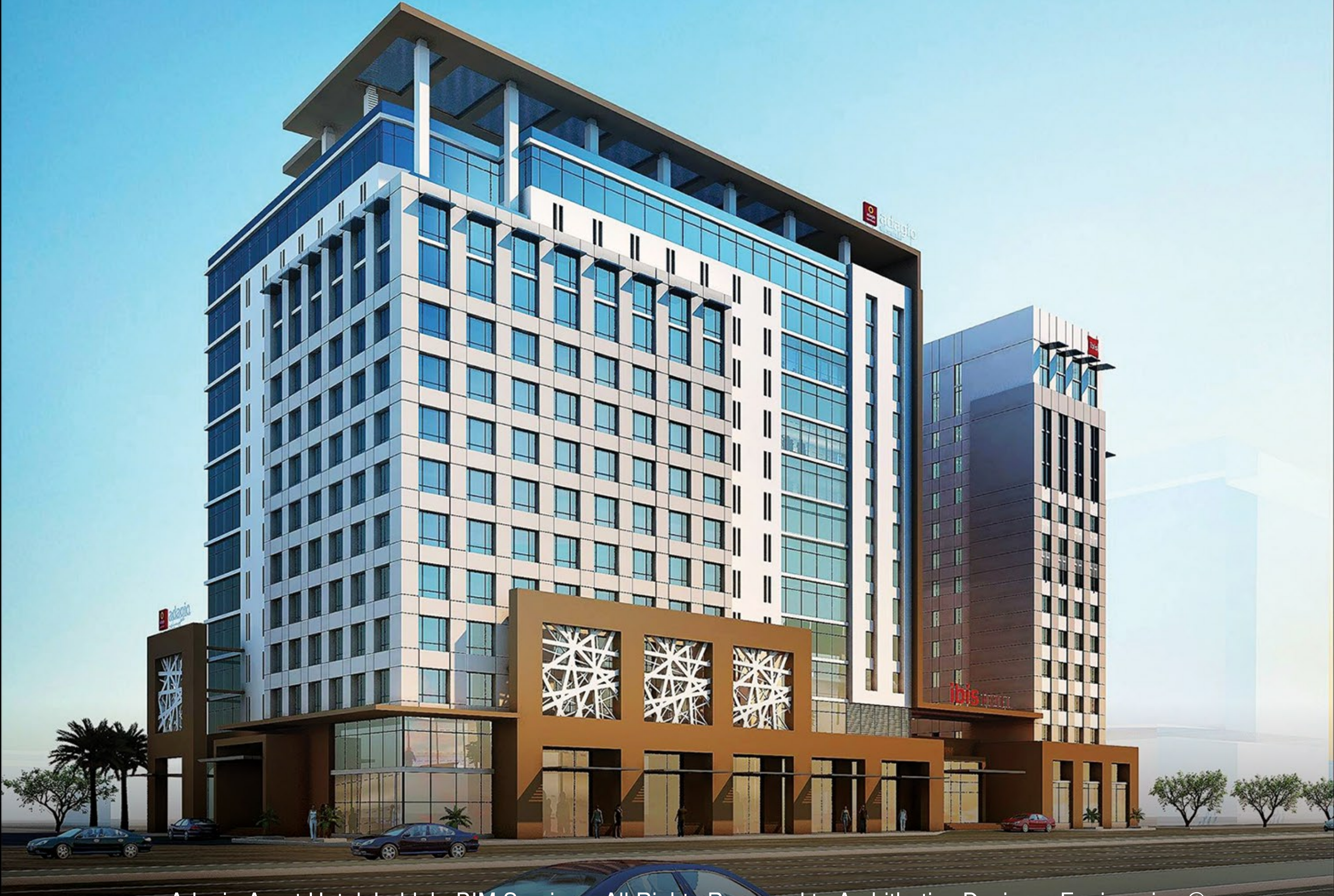
Adagio Apart Hotel,Jeddah, BIM Services. All Rights Reserved to Archithetics Design + Engineering ©
